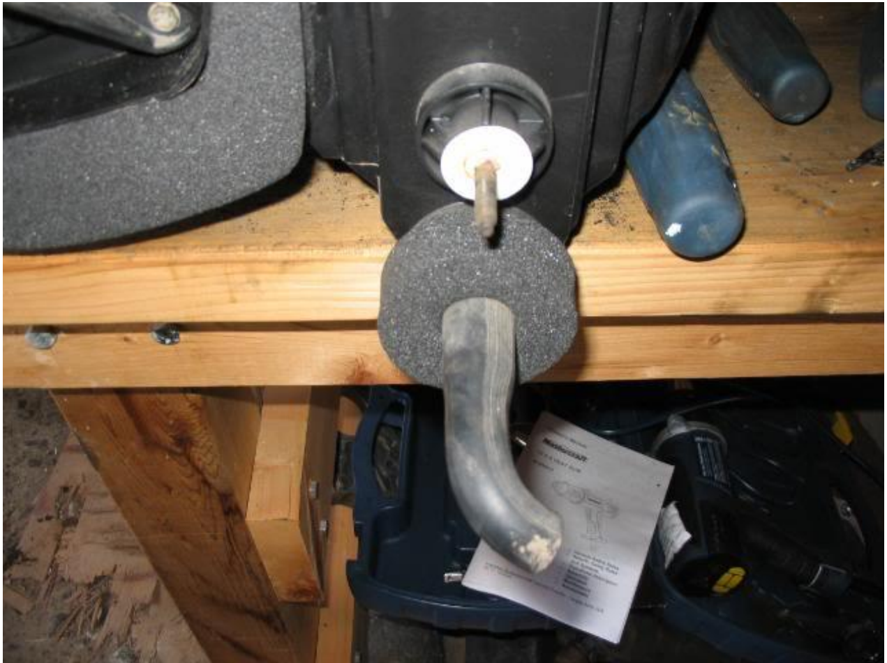
HVAC box reinstalled:
